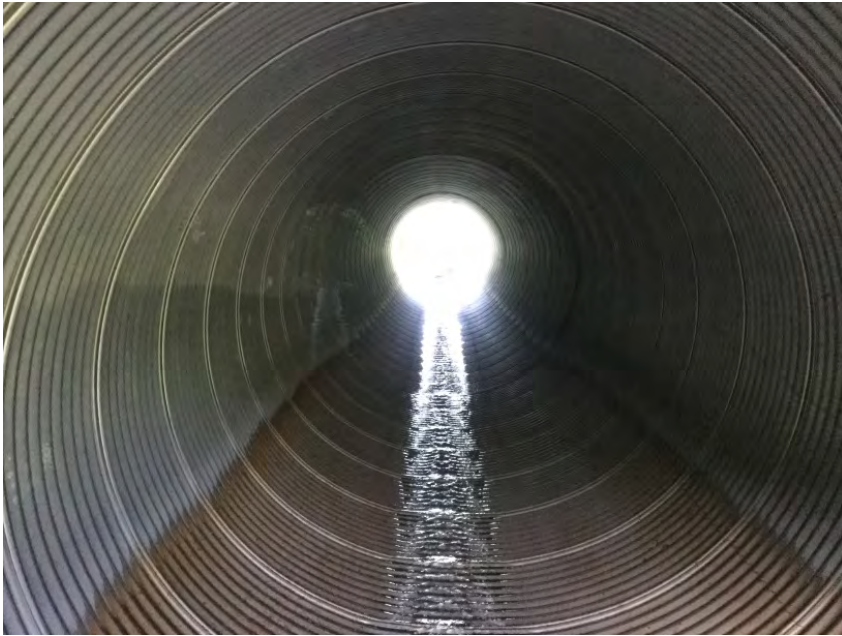
Looking through culvert from inlet
